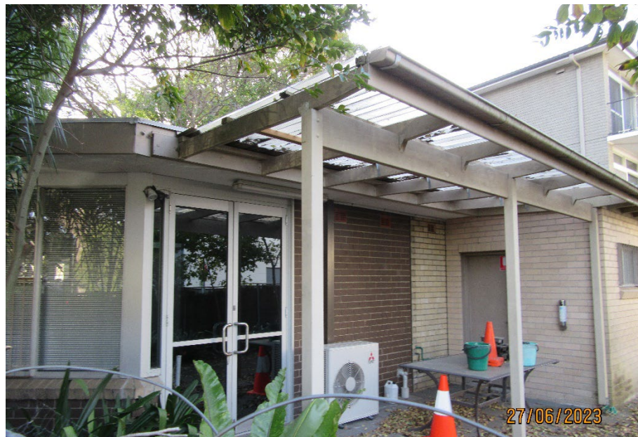
19 Pergola and laundry (at right) facing Allen Lane.
