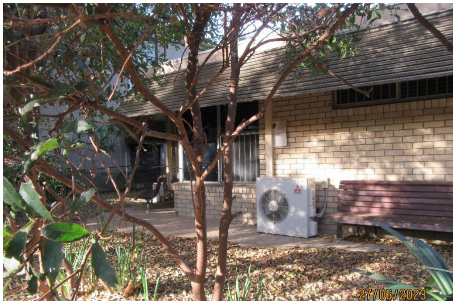
16 Western side of the building, showing the lightweight metal awnings installed to shade windows and details of fenestration, on this side of the building.
